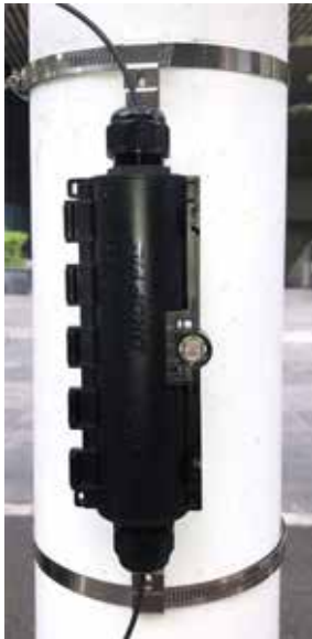
Pole Mount Installation
